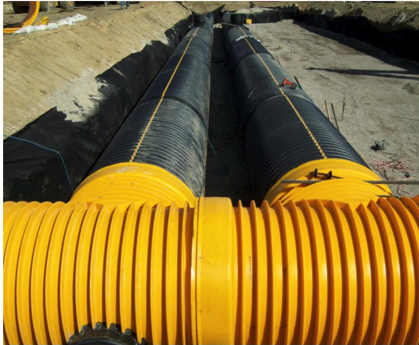
Figure 6.9: Underground enclosed detention chamber (courtesy of Prinsco)
