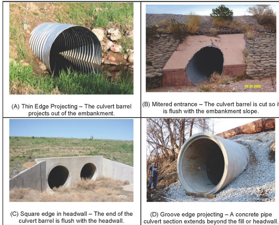
Figure 6.2: Common culvert entrance configurations (FHWA HDS No. 5 1985)
